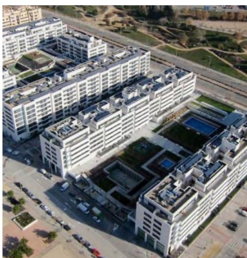
The PAUs reproduce the strategy of the Castro Plan , creating homogeneous neighbourhoods in the periphery, but with better construction quality. In recent decades, a new belt of commuter quarters for different social strata has shaped the contemporary periphery of Madrid. PAU of Arroyo del Fresno, Fuencarral-El Pardo. Source: Publicidad de Construcciones Amenabar, 2022.
