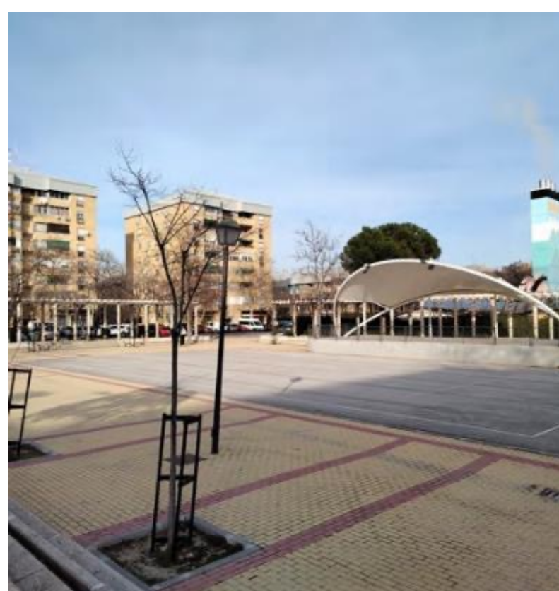
After a long struggle by local residents, Orcasitas was demolished in 1984 and replaced by a new neighbourhood of blocks with better quality housing and improved infrastructure and urban services. It is a remarkable case because it is the first time that effective citizen participation in the design of the environment has taken place. Plaza de la Asociación de Orcasitas , Usera , 1986. Photo: Eulalia Portela , 2020. Courtesy of the author.
