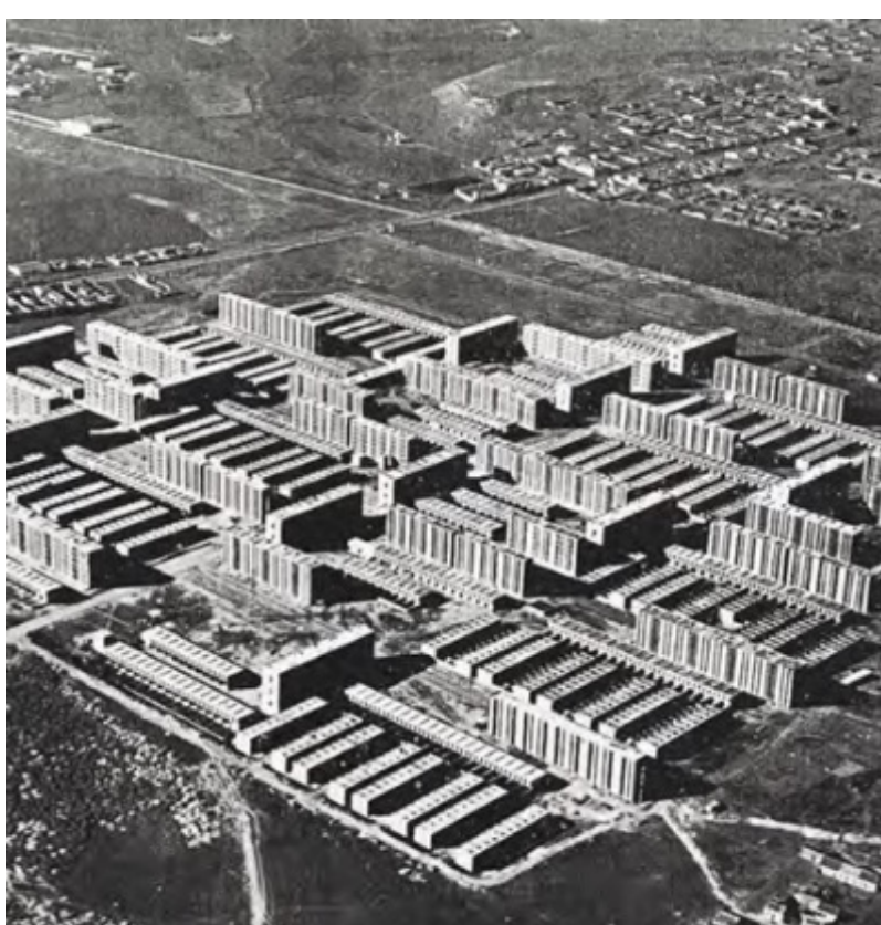
Orcasitas is a good example of the Neighbourhood Redevelopment Plan. Designed in 1957, the poblado had an experimental character, praised for its avant-garde conception, but the low quality of the materials, the construction flaws and the lack of geotechnical studies caused serious pathologies in the buildings. Poblado Dirigido de Orcasitas , ca. 1960. Source: Servicios Aéreos Norte , Blog Urbanidade , 46, 2011.
